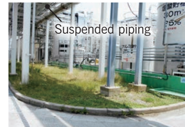
Execution of the pollution prevention work
