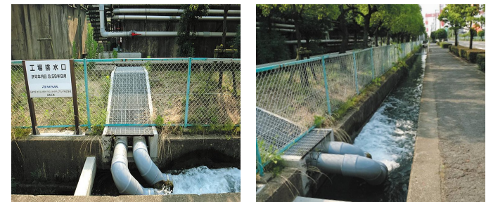
Visible factory wastewater pipes
