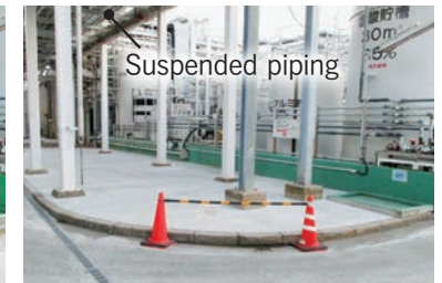
After the pollution prevention work
